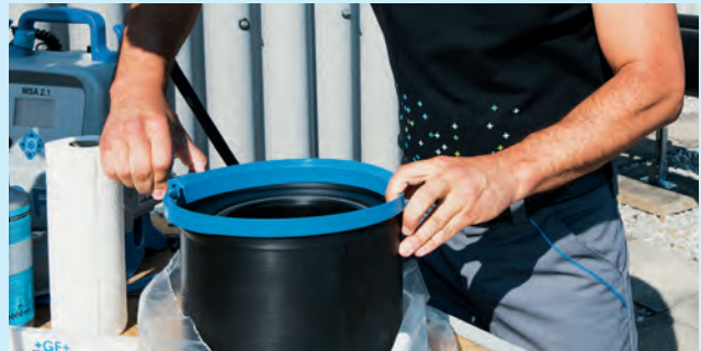
Place the mounting aid on the fitting. Stretch the sealing lip pressing the handles together.
