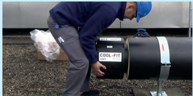
Slide-on the shrink sleeves and push the pipe ends up to the stop into the electrofusion coupler.
